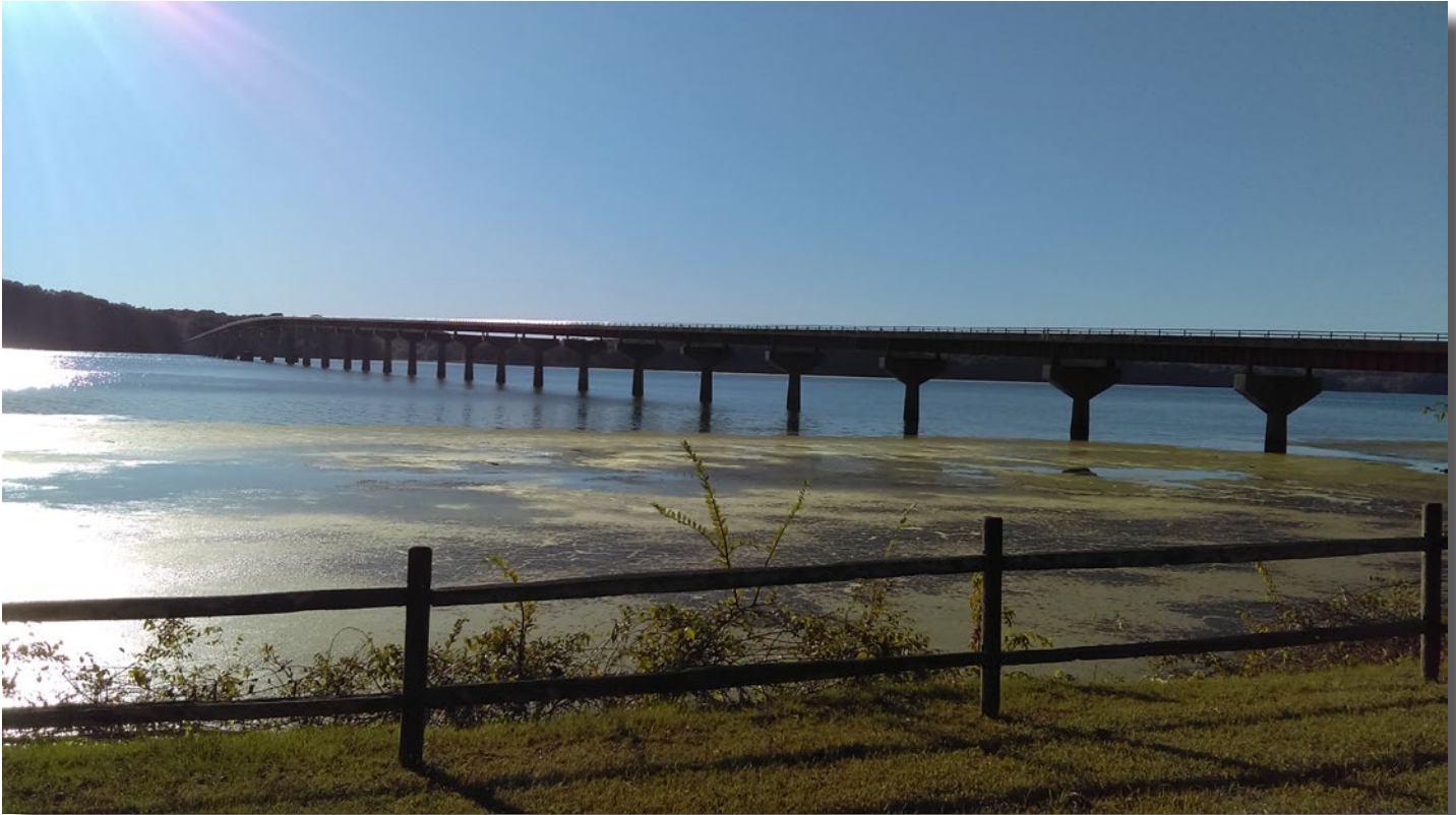
The Tennessee River — A view of the Natchez Trace Parkway Bridge over Pickwick Lake on the Tennessee River in northwest Alabama, October 2019.
