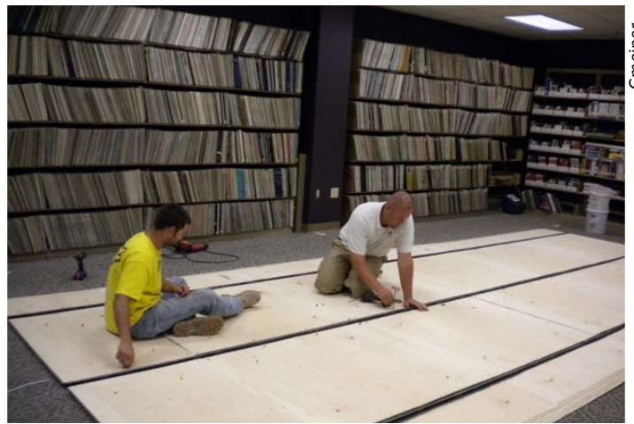
Construction of the Compact shelving...the laying of the platform and tracks. We chose to keep LPs on the peripheral wall shelves. We learned that the weight load would have been too great if we incorporated those into the center.
