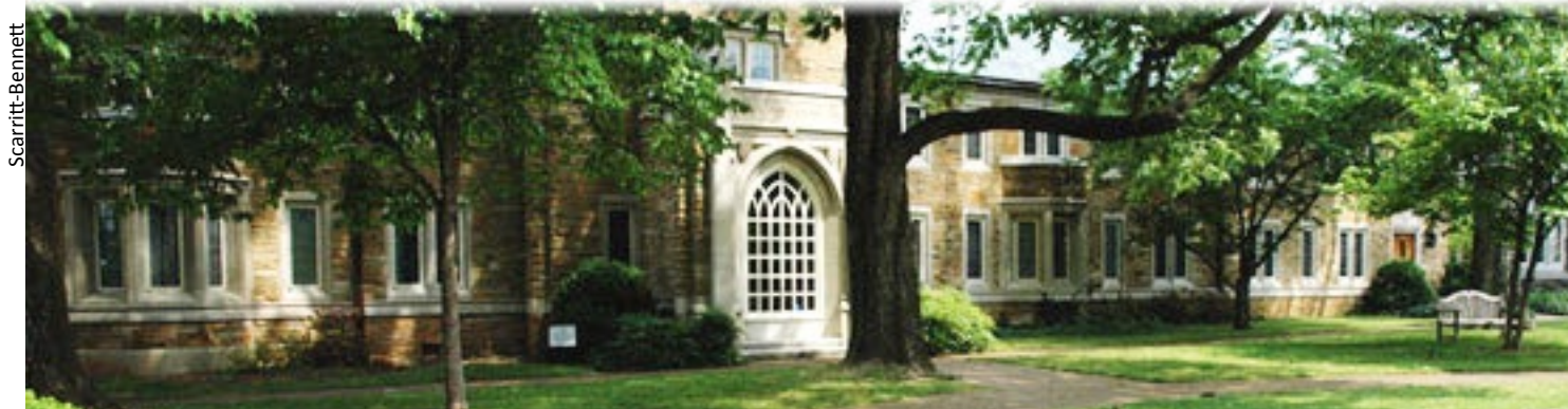
Scarritt Bennett Center — Gibson Hall
